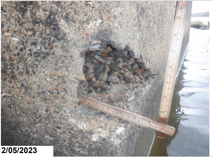
Bent 56, column 2: Spall with exposed rebar on the northeast corner, 25% section loss to the reinforcing steel. 2SF CS3
