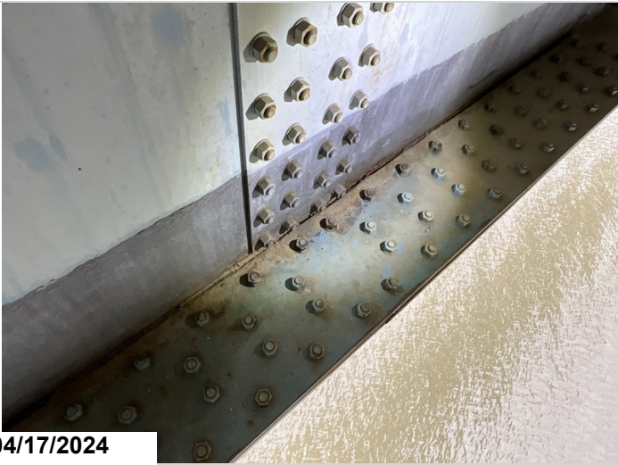
Span 56, girder 1, right, splice 1: Has active corrosion with up to 1/8th of section loss for the length of the splice. 6LF CS3
