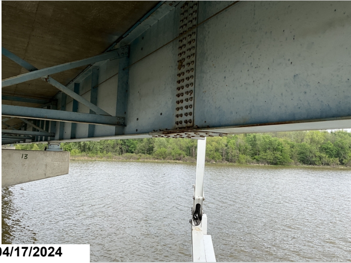
Minor pack rust at several splice locations.
