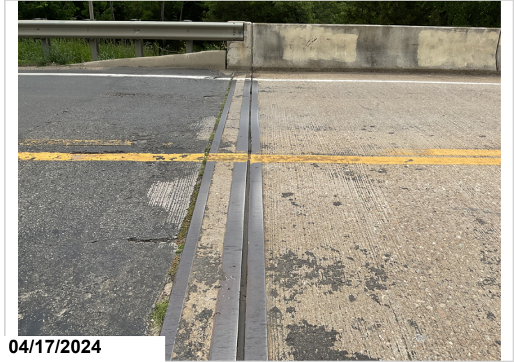
Typical joint condition over abutments.
