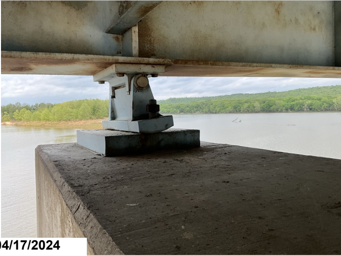
Bent 50, bearing 1: Is near full rotation at 69 degrees. 1EA CS3
