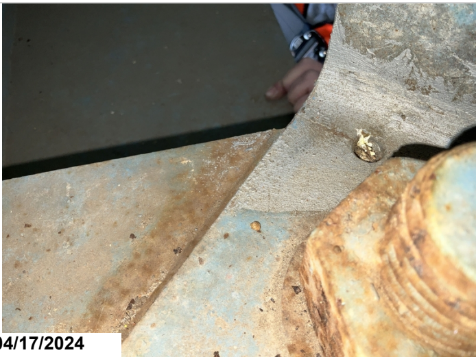
Span 56, girder 1, floor beam 1: 1" crack in base plate at lateral brace connection has been arrested. 1LF CS2
