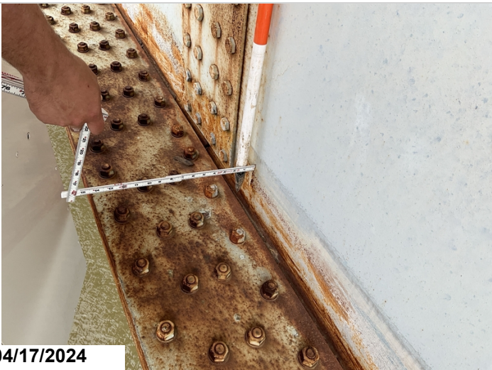
Span 56, girder 1, 1st splice: Out of plane bending of web. The middle section of the web measures 3/4" out and increases to 1" at the bottom. 6LF CS2
