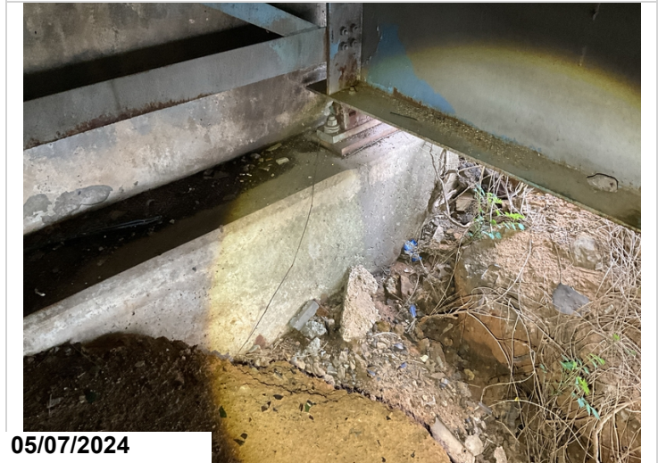
Abutment 1, left: Scour exposing 3' of the cap face vertically. Scour begins at the left edge and travels toward the center for 8'.
