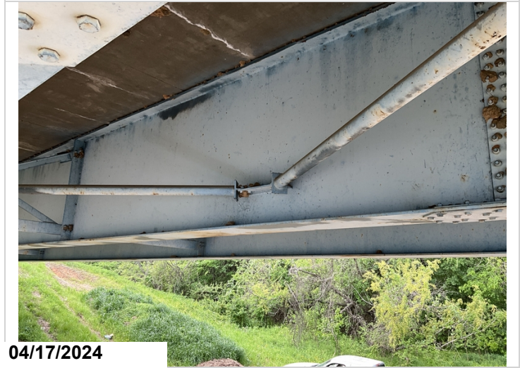
E details: lateral bracing to girder web welds approach spans.
