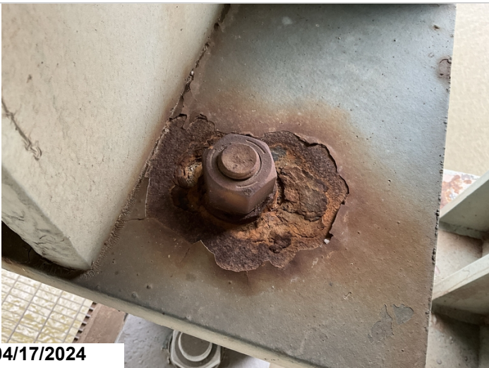
Span 56, Bent 56, girder 2, left: The bearing connections have section loss around the bolt hole. 1/8" typical. Girder 1 at this bent is similarly deteriorated. 2LF CS3
