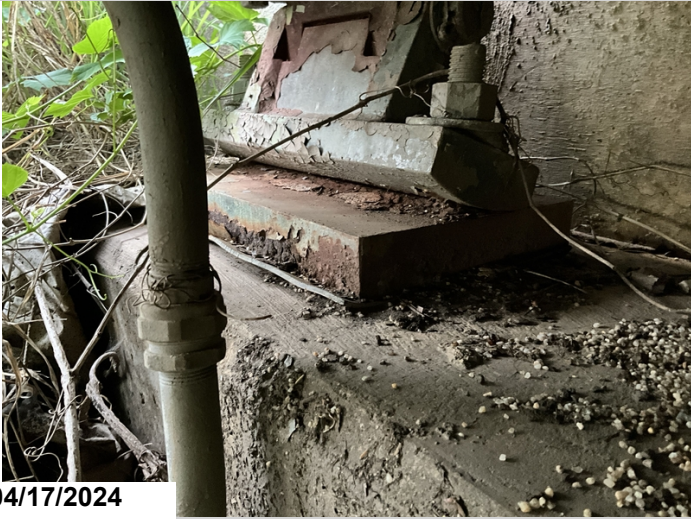
Typical corrosion in bearings at the abutments. CS3
