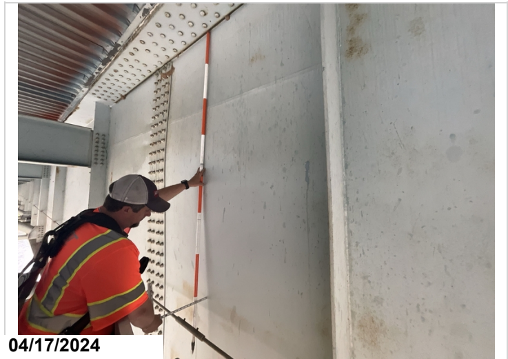
Span 56, girder 2, left, splice 1: Has up to 1.5" of out-of-plane bending to web. 5LF CS2
