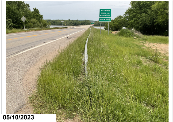
Approach Railing, right side, beginning of structure: has minor collision damage. CS2
