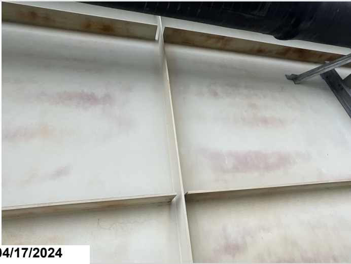
E details. Longitudinal stiffener terminations. Sufficient gap between the longitudinal and vertical stiffeners.
