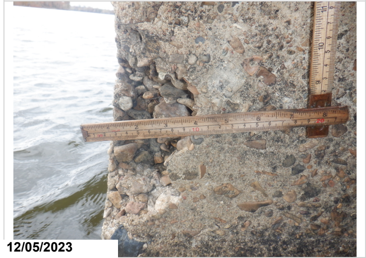
Bent 56, column 2: Spall on the southeast corner. 2SF CS3
