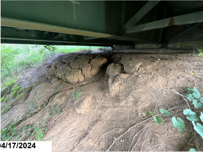
Abutment 2: has minor erosion. No exposure of the face.
