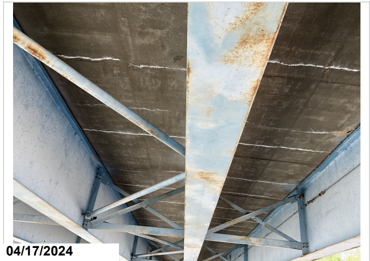
Approach spans: have an average of 7' spacing for efflorescence. 17226SF CS2
