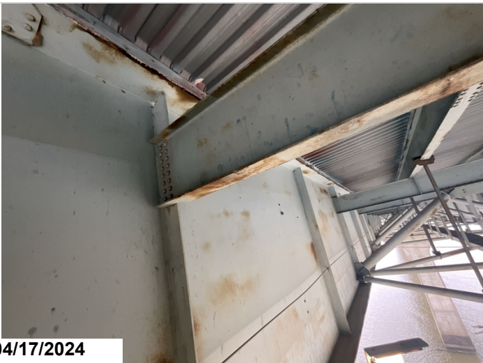
Typical corrosion along the top flange of girders. CS3
