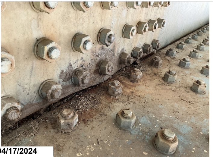
Span 57, girder 2 left, 3rd splice: Has a bulge at the bottom of web splice plate. 1LF CS2
