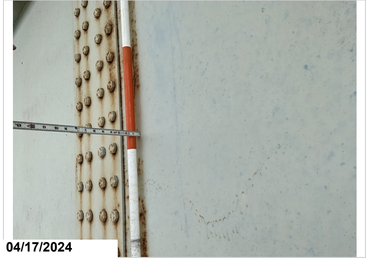
Span 56, girder 1, 1st splice: Out of plane bending of web. The middle section of the web measures 3/4" out and increases to 1" at the bottom. 6LF CS2
