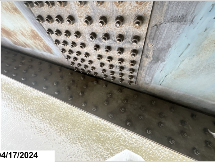
Span 56, girder 1, right, 3rd splice: Has minor section loss at splice connection up to 1/8". 1LF CS3
