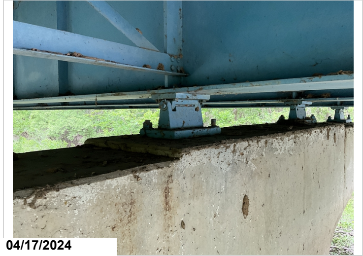
Span 28, bent 29, back: Bearing 2 has its right nut missing. 1EA CS3
