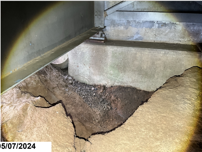
Abutment 1: has a scour hole on the right side that exposes the entire abutment face for 10', beginning at the right edge and traveling toward the center.
