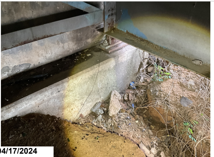
Abutment 1, left: Scour exposing 3' of the cap face vertically. Scour begins at the left edge and travels toward the center for 8'.
