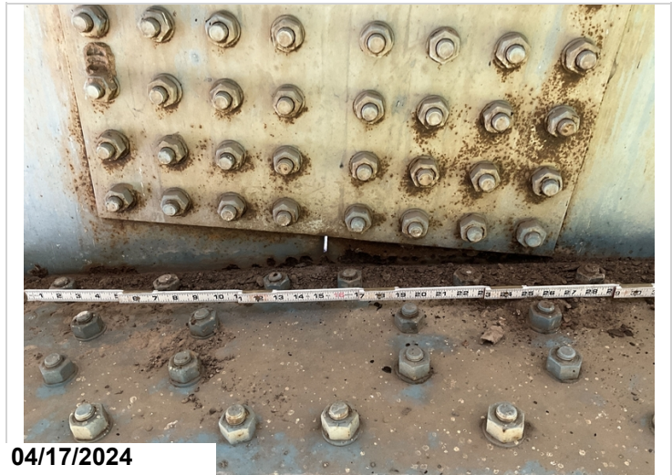
Span 58, girder 1, right, splice 1: Has 1/16" x 28" section loss to the lower web between the web and bottom flange splice plate. 3LF CS3
