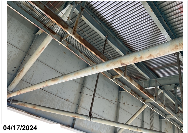
Span 57, lower chord of floor beam 8: typical failing paint and corrosion. CS2
