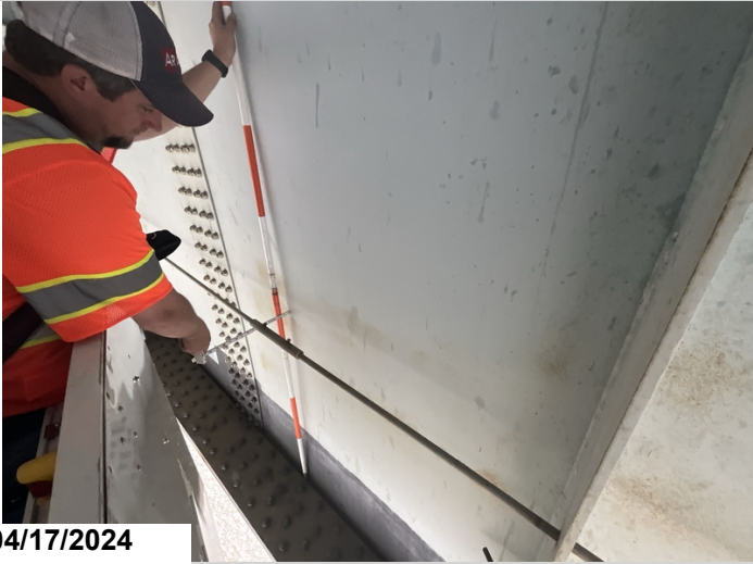
Span 56, girder 2, left, 1st splice: 1.5" out of plane bending to girder web. 5 LFCS2
