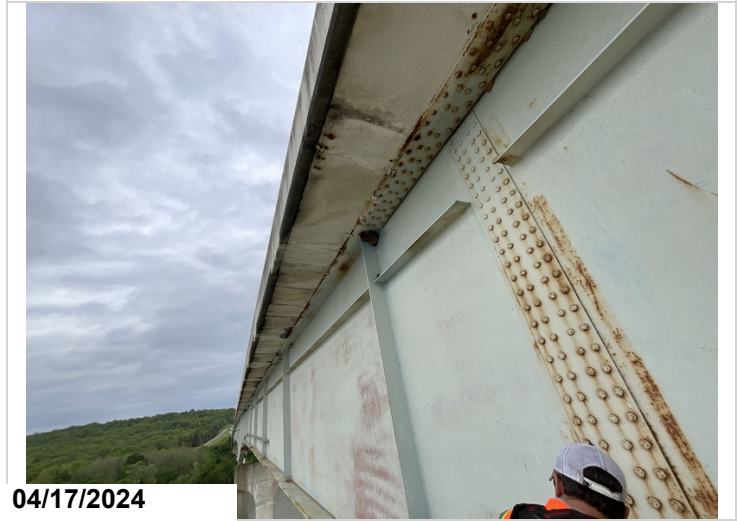
Span 56, left, Overhang: has cracking at 3' spacing with heavy spalls. 2SF CS3
