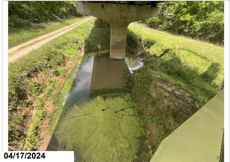
Span 20: Has a large scour hole.
