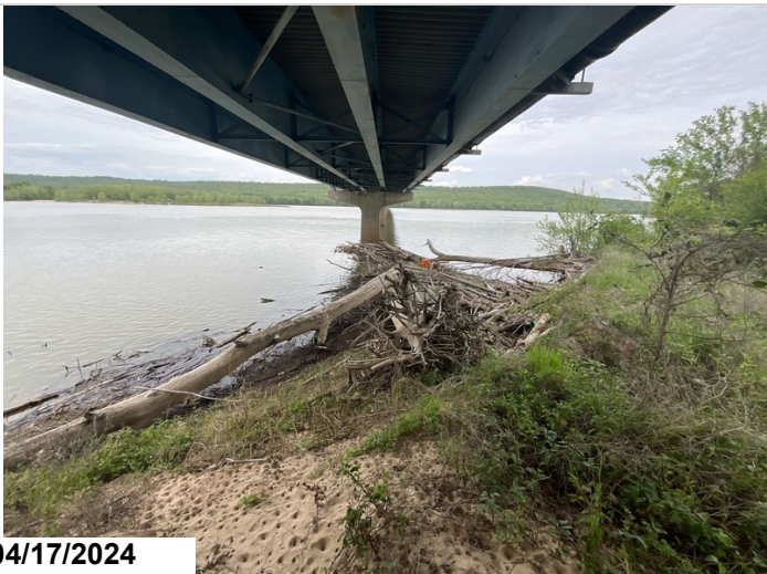
Span 41: Has debris and cutting of the channel bank.
