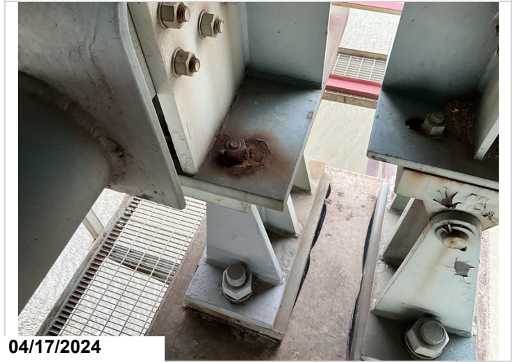
Span 56, Bent 56, girder 2, left: The bearing connections have section loss around the bolt hole. 1/8" typical. Girder 1 at this bent is similarly deteriorated. 2LF CS3
