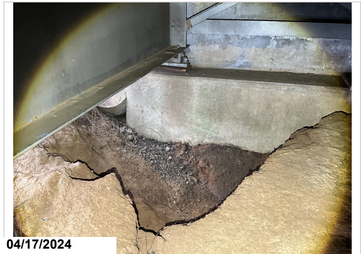
Abutment 1: has a scour hole on the right side that exposes the entire abutment face for 10', beginning at the right edge and traveling toward the center.
