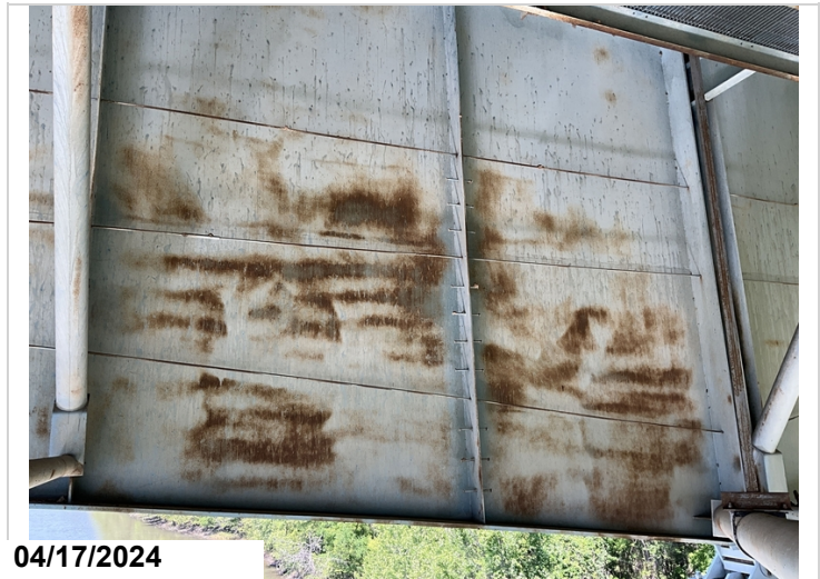
Span 57, pier 58, girder 1, right: Typical paint system failure and surface corrosion. CS3
