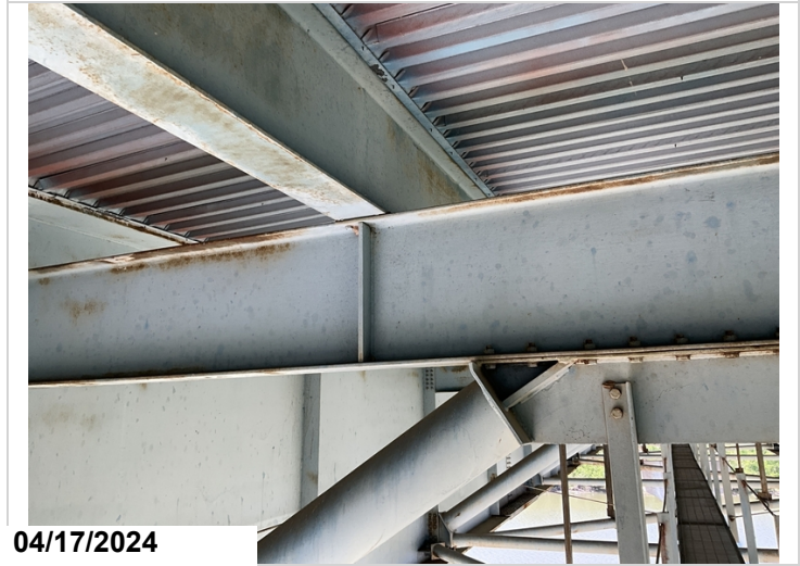
Span 56, floor beam 2: typical surface corrosion to floor beams. CS2
