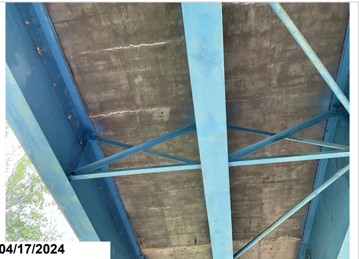
Span 33, bay 1, Diaphragm 4: There is a spall to the undersurface with exposed rebar. 1LF CS3
