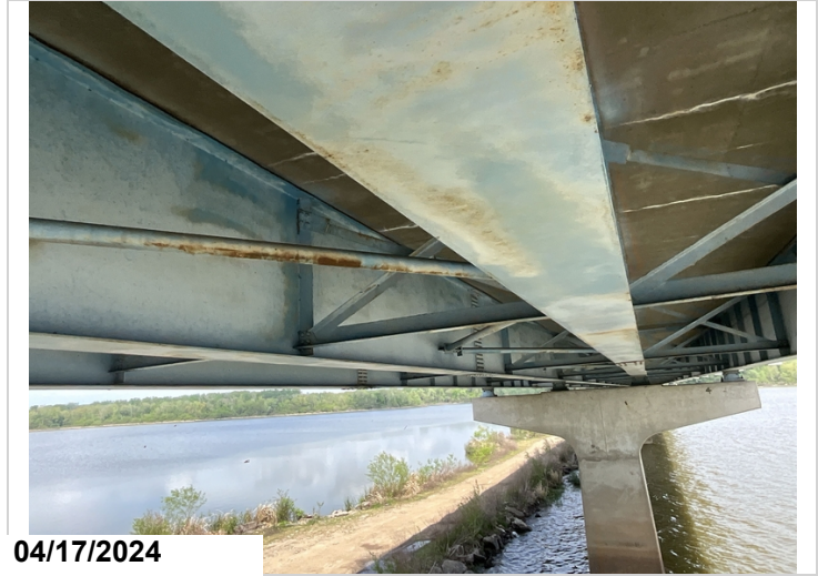
Typical paint condition approach span girders.
