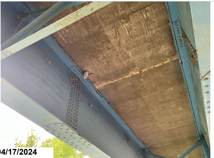
Span 39, bay 1, 1st splice: Has spalls with exposed rebar. 2SF CS3 There are delaminations adjacent to this area. 2SF CS2
